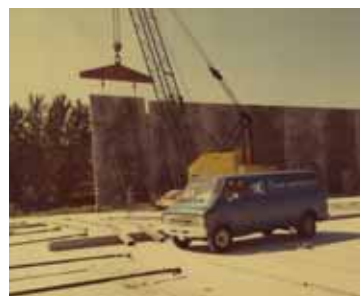
Innovative tilt-up industrial construction method / 1960s
